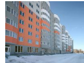
Residential Building in Verhnaya Pyshma, Sverdlovsk Oblast, Yekaterinburg, Russia 2014
