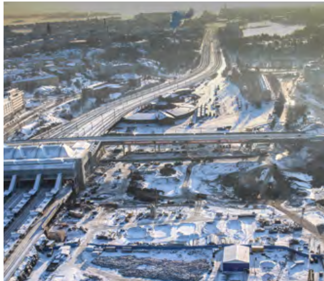
Excavation work on the first phase of the Tripla project—the parking facility—was underway in Central Pasila in December.
