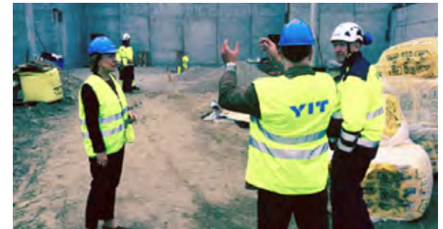
It is important for customers to stay up-to-date on progress of construction. In the photo, head supervisor Markku Lindholm shows visitors around the As Oy Tampereen Kristalli site.
