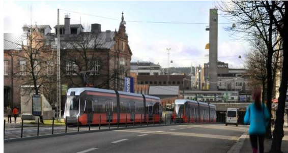
Tampere light rail alliance project
