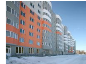
Residential Building in Verhnaya Pyshma, Sverdlovsk Oblast, Yekaterinburg 2014
