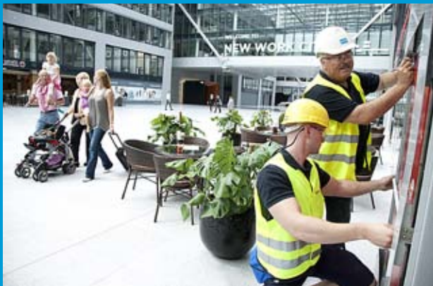
Manfred and Florian are making sure that the fire safety is in order.
